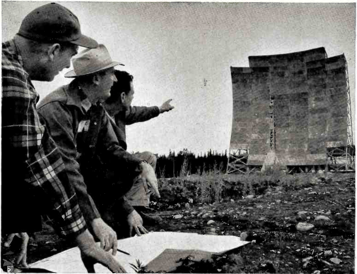
Screen-like parabolic antenna is used in dramatic new "over-the-horizon" transmission technique on White Alice. Giant antennas like this, built to Bell Laboratories design, receive and transmit signals beamed from more than 150 miles away and scattered back to earth by the troposphere.
