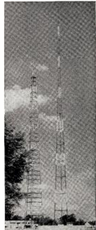
WKBN-TV Truscon Self-Supporting Tower 539-Feet Tall
