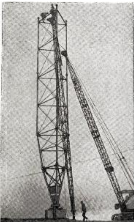
Construction close-up on new 1282-foot Truscon Triangular Guyed Tower for WWTW in Cadillac, Mich.
