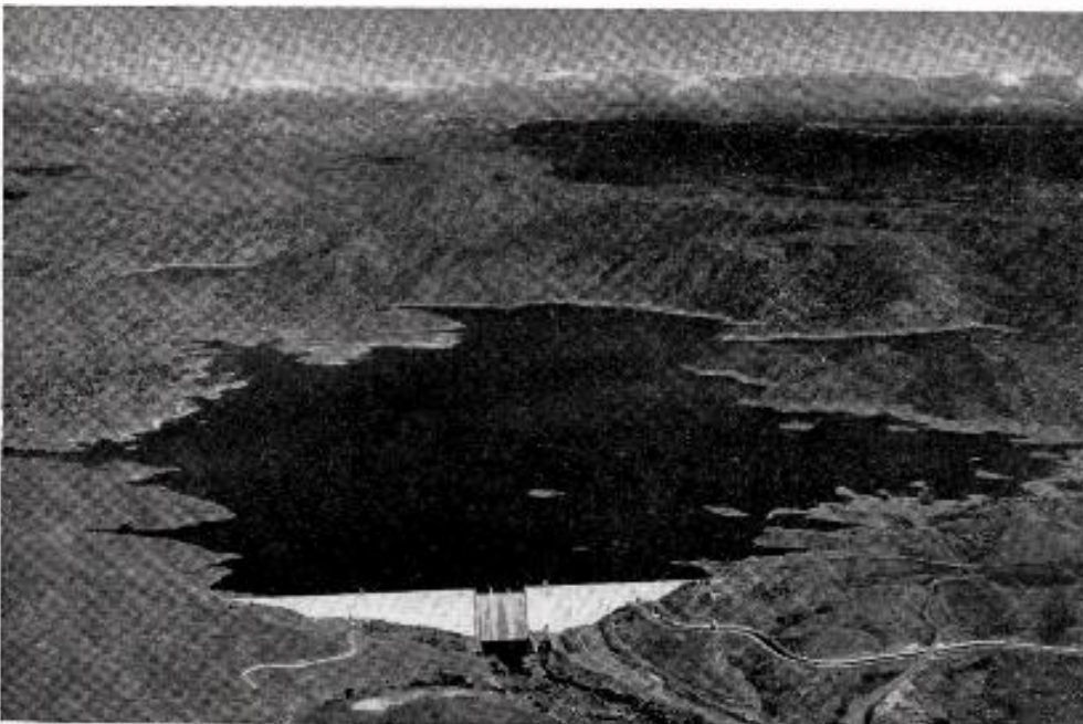
FRIANT DAM: The world's fourth largest, it supplies water and power for the San Joaquin Valley. A newer dam, Pine Flat, is in operation just east of Fresno.
