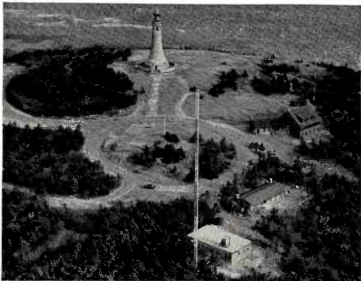
Air view of the summit of Mt. Greylock with the WMGT transmitter building at the bottom of the picture and the town of Adams, Mass. in the distance. The tower in the center of the picture is a War Veterans Memorial familiar to all living within a 100-mile radius of this pinnacle 3700 feet above sea level.
