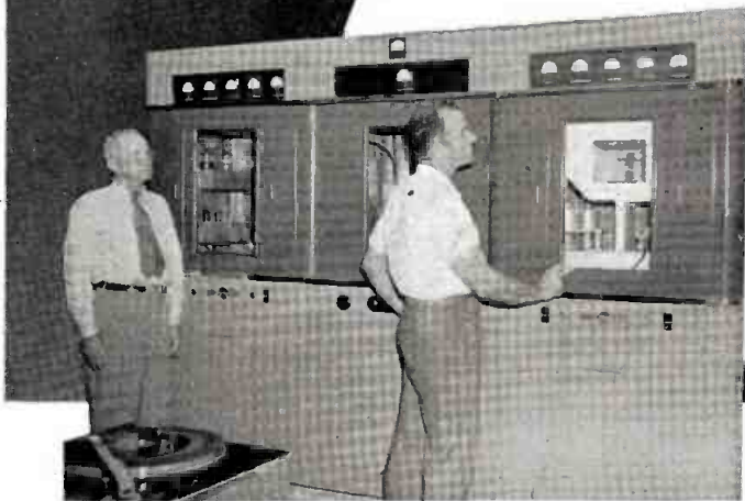
Hugh J. Fite (left) and Charles B. Tucker, Chief Engineer, with WERH's new Collins 21E 5 kw transmitter.
