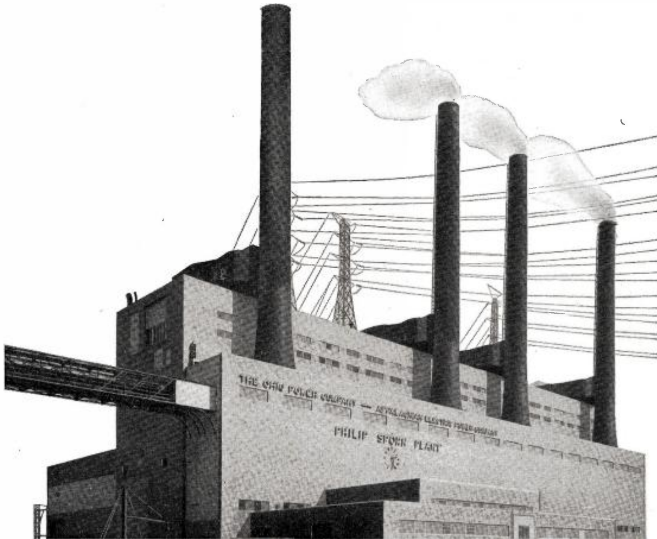
This $66,000,000 steam-electric generating station, the Philip Sporn Plant at Graham Station, W. Va., is among the world's largest and most modern. Its output capacity of 600,000 kilowatts supplies power for major industries and industrial communities throughout WSAZ-TV's 114-county area.
