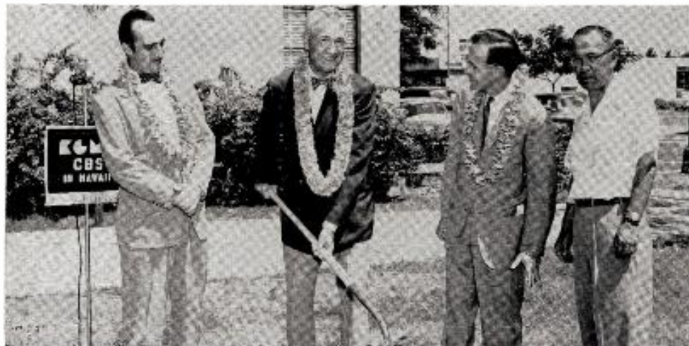
HAWAIIAN Broadcasting System executives breaking ground for the new $100,000 KGMB-AM-TV Honolulu Radio-TV Center, to be located adjacent to the present KGMB building and which will house a 5,400 sq.-ft. TV studio, are (l to r) Dan Hunter, chief engineer; J. Howard Worrall, president; Wayne Kearl, assistant general manager, and Akiyoshi Hayashida, head of KGMB's Japanese Dept.
