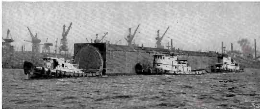
One of the 300-ft steel tunnel sections starting on its voyage down Chesapeake Bay. Seven of these sections were fabricated at Bethlehem's Sparrows Point shipyard, near Baltimore, and were towed to the tunnel site at Norfolk, Virginia.
