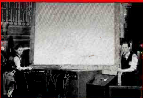
First Theatre Television. In May, 1930, Dr. Alexanderson produced a picture 7 feet square on a screen in Proctor's Theater, Schenectady. Receiver used a light cell developed by Dr. August Karalus.
