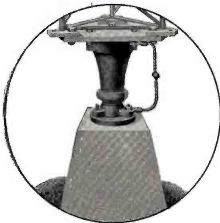
Base insulated central pier showing "Most-Base" or "Pivot" type base insulator with Spark-Gap.
