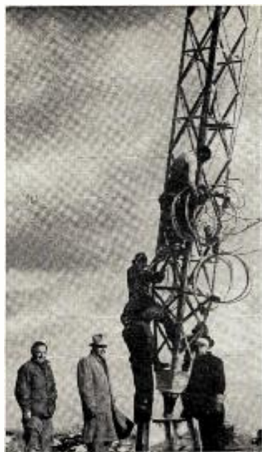
WICH Norwich, Conn., increases coverage by an estimated 40% with a 357-foot-high half wave radiator. In the foreground are (l to r) Alexander Dubenetsky, WICH chief engineer; John Deme, president and general manager of the station, and John J. Hoke, president of Consolidated Tower Construction Co., Petersburg, Va.
