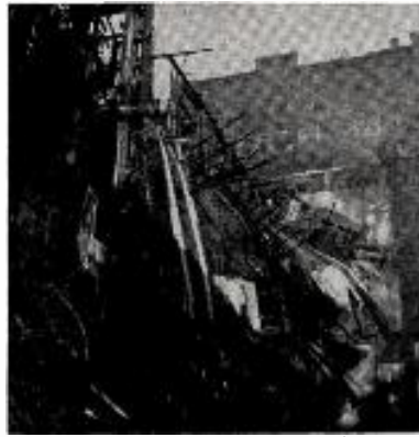
This is how the interior of the Ridpath Hotel looked from the KXLY "fire door."
