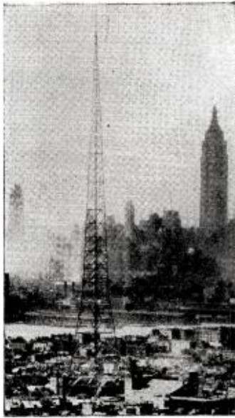
WITH part of New York City skyline in background, new WOR-TV New York transmitter rises off Palisades (foreground) at North Bergen, N. J. Site of the transmitter is 240 ft. above the Hudson River, and the 760-ft. tower rises to within 200 ft. of Empire State Bldg. height (in background, r). Station plans to go on the air on Channel 9 (186-192 mc) in late summer.
