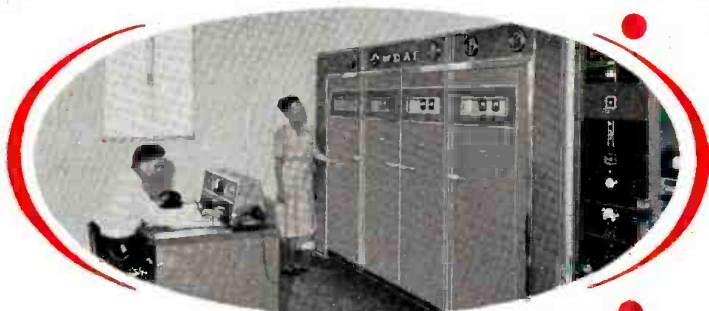
WDAE—TAMPA —Owned and operated by the Tampa Daily Times, the city's oldest station has been on the air since 1922. In recent complete modernization program, WDAE officials selected the General Electric 5 kw AM transmitter (above).
