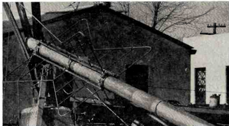
HERE is the top segment of the six-bay super-turnstile antenna of WTVR (TV) Richmond, Va., being lifted into place atop the new 417-ft. tower. With completion of the antenna the station will operate with its full authorized power of 12.16 kw visual, 6.4 aural.
