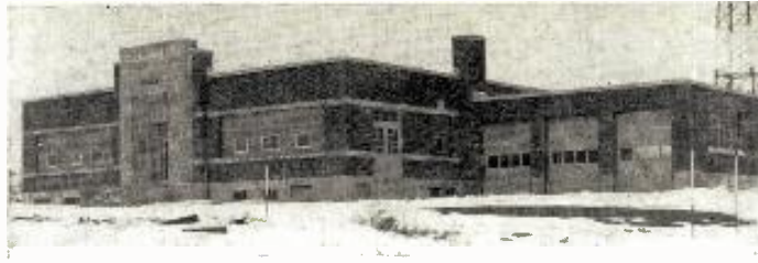
WTAG's transmitter building.
