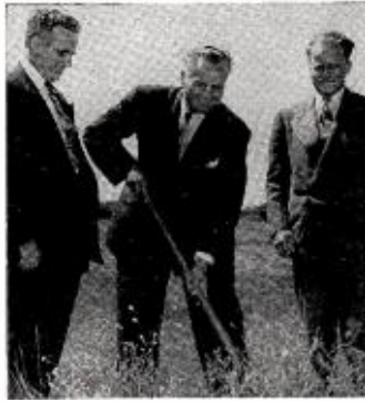
GOVERNOR Luther W. Youngdahl of Minnesota (center) is shown breaking ground for the transmitter of KEYD Minneapolis, new 5-kw daytime outlet which expects to be on the air by Oct. 1. Observing are Lee L. Whiting (l), manager, and Harold Winther, commercial manager.
