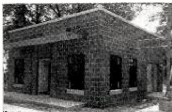
View of transmitter building and antenna base of WPAY-FM.
