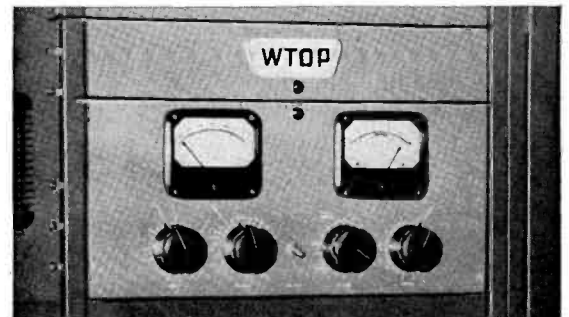
G-E Limiting Amplifier at the 50,000 watt transmitter of WTOP, Washington, D. C.
