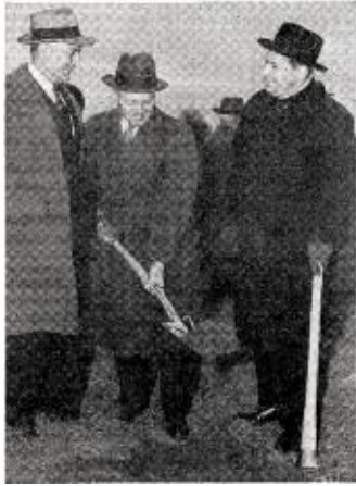
ANOTHER SHOVEL hits the dirt as officials of WFIL Philadelphia signal start of construction of the station's new 5,000 w transmitter in Whitmarsh Township. Roger W. Clipp, WFIL general manager, handles the shovel, while Louis E. Littlejohn (l), chief engineer, and Walter H. Annenberg, publisher of The Philadelphia Inquirer , owner of WFIL, give advice from the sidelines.
