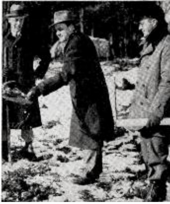
GROUND IS BROKEN for 450-ft. tower of WFMR New Bedford, Mass., Jan. 7 by William R. Hutchins, WFMR manager and chief engineer. With Mr. Hutchins are William Tallman (l), architect for the station, and Stanley S. Emery, Jr. WFMR engineer.
