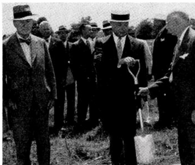
TURNING THE FIRST SPADE for the new Princeton Laboratories of RCA, a three-story structure with a one-story wing on a 25-acre tract, are high officials of the company, who dedicated the building to the application of radio and electronics to national defense. First spadeful was turned by Otto S. Schairer (right), vice-president in charge of the RCA Laboratories. At left is Maj. Gen. James G. Harbord, chairman of the RCA board, and in center is David Sarnoff, RCA president. Forty company directors and executives were present for the ceremony.
