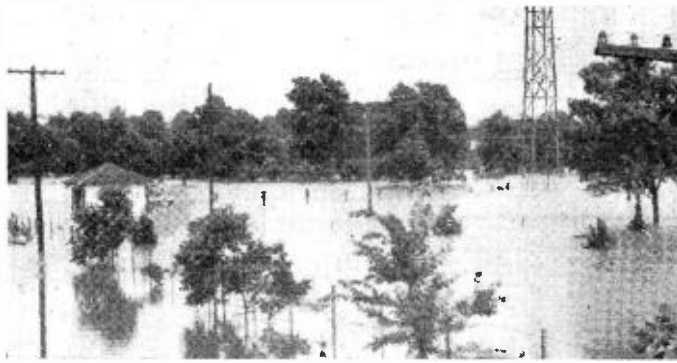
WATER EVERYWHERE, the most in 15 years, inundated the transmitter site of KHBG, Okmulgee, Okla., throwing the station off the air 45 hours. Water was 2½-feet deep in the transmitter house at left and the tuning house was completely submerged.
