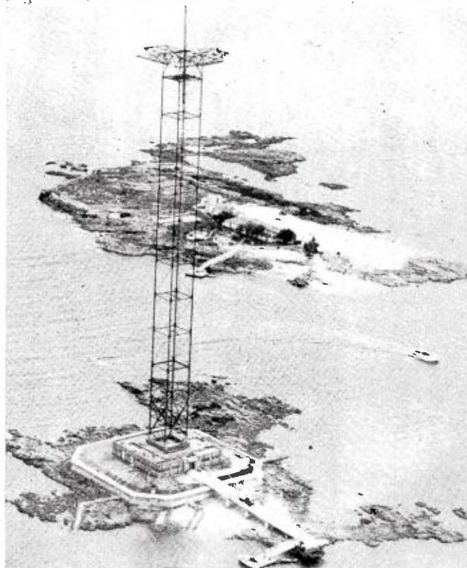
A MILE OFF New Rochelle, N. Y., on tiny Pea Island in Long Island Sound, the new transmitter of WABC, New York, has been completed, and will be used for broadcasts early this fall. The 300-foot tower rests on a concrete platform constructed by WABC engineers as the island itself was nothing more than a group of jagged rocks barely projecting out of the Sound at high tide.
