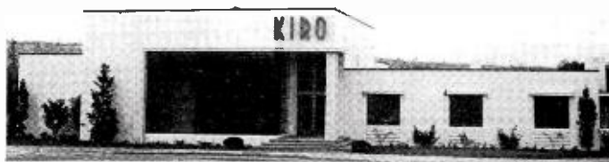
NEW 50 KW. PLANT of KIRO, Seattle, placed in operation this week, is located on an island in Puget Sound, halfway between Seattle and Tacoma. Its two 526-foot towers are described as the only 50-kw. directional west of the Mississippi.
