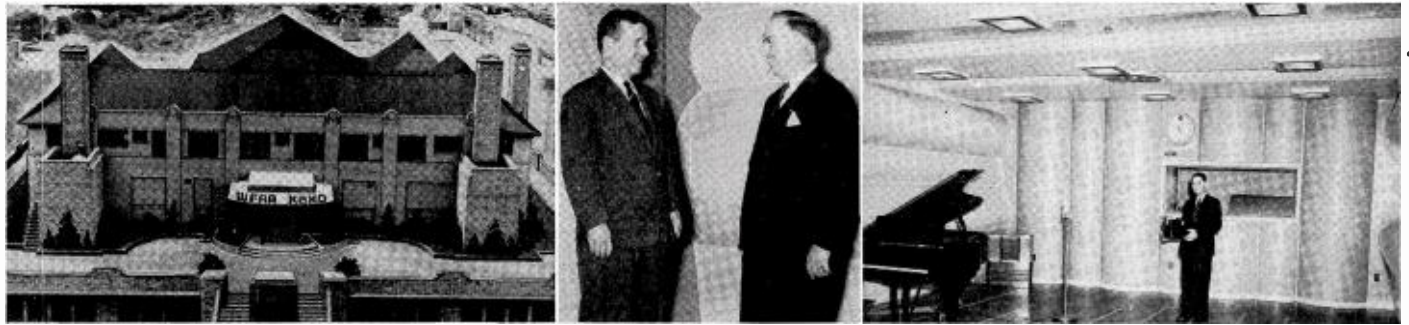
PENTHOUSE STUDIOS of WFAA-KGKO atop Dallas' Santa Fe Bldg. incorporate novel and advanced techniques. At left is the two-story penthouse, which contains five studios and control rooms and 30 other rooms, including executive offices, news, recording and client rooms. In center photo J. M. Moroney (left), vice-president and radio supervisor of the Dallas News , owner of WFAA and co-owner (with the Fort Worth Star-Telegram ) of KGKO, is shown with Martin Campbell, managing director
