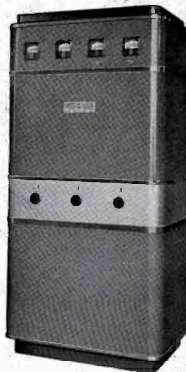
RCA Antenna Phasing and Branching Equipment at WLAW, Laurence, Massachusetts
