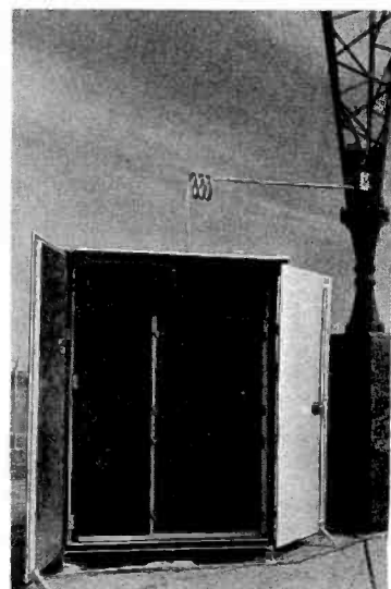
Western Electric antenna coupler equipment for the 50 KW transmitter.
