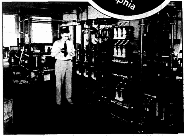
The mercury-vapor type rectifier shown in the unit above was designed and manufactured by Westinghouse for its new Philadelphia Station. It measures 6 by 6 feet and is only 3½ feet deep. Although small in size, it contains a 17-amp., 12,000-volt main rectifier, a 2.5-amp., 3000-volt intermediate rectifier and a 1500-volt bias rectifier. In addition, it contains circuits to reduce telephoning line interference. D. C. output ripple content is less than 1/10 of 1 per cent.
