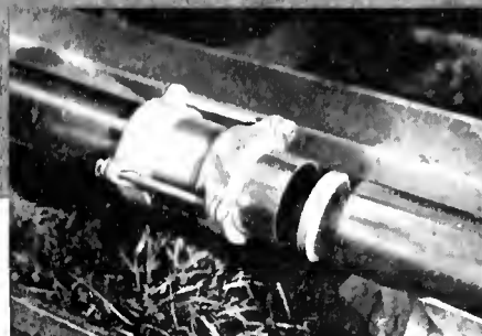
Above: Locking insulator located at center of line allows two-way expansion. Solderless connectors provide gas-tight joints.
