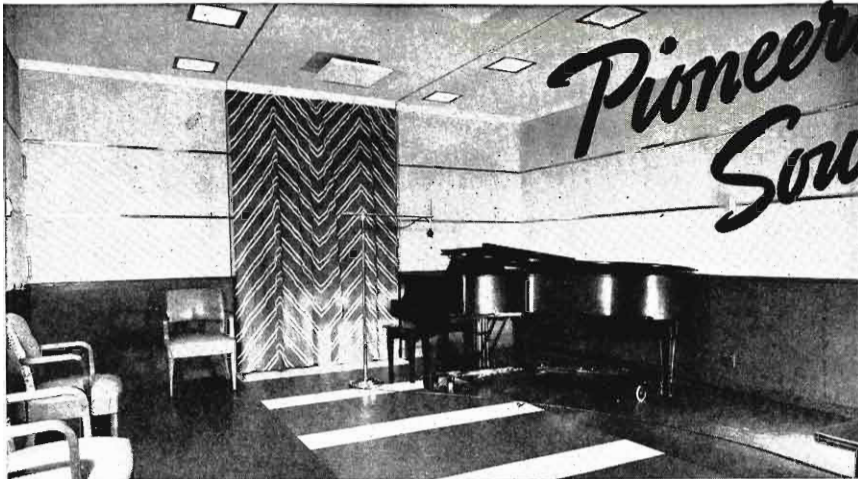
One of the new WWJ studios treated on walls and ceilings with J-M Sound-Control Materials and isolated from the rest of the structure by the J-M system of sound isolation. Note the adaptability of the material to the modern decorative style.
