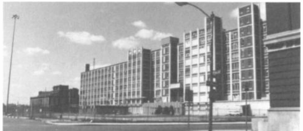
Figure 6. These other "old" GE/RCA/VTMC buildings in Camden are likely targets for demolition. However, building #17, seen in the extreme right corner of the photo, will be preserved.
