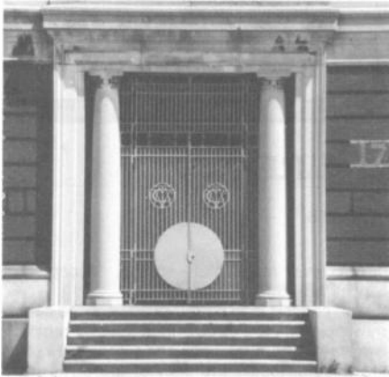
Figure 5. Wrought iron gates with "VTMC" (Victor Talking Machine Co.) superimposed in the ironwork.
