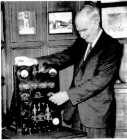
Figure 6. Lee de Forest with his early vacuum tube transmitter, which superceded the Arc Fone technology.
