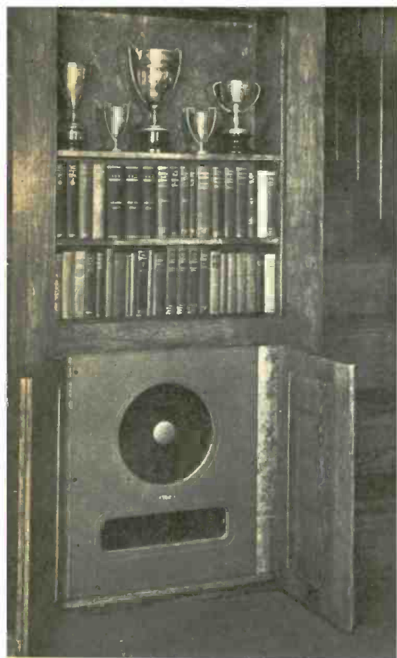
Fig. 1. One of the several remotely-located Jensen 15-inch Peridynamic speakers. A 500-ohm line is run from each of the several speakers to the main amplifier in the basement.
