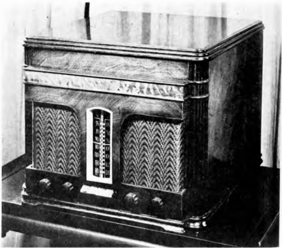
This 6-tube superheterodyne table combination in mahogany cabinet has an automatic record changer and push-button selection.
