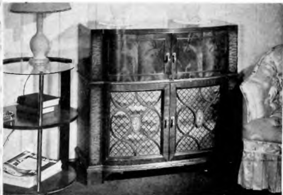
Console of Sparton features radio-phonograph with automatic player, FM-AM, short-wave.
