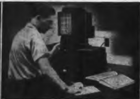
To constantly improve metals for trumpets Conn uses latest scientific tools, such as $10,000 spectroscope which detects metals in an alloy in as small amounts as one part in one million.
