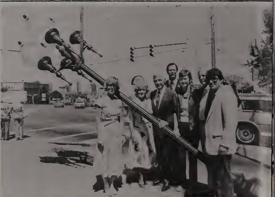
ROWSCAPING -- Mayor Richard Fulton and members of the Music Row Redevelopment Steering Committee lend a hand in the installation of the first streetlight for the current plan to improve the appearance of Nashville's music industry neighborhood. Pictured are: Mary Anne Harwell, Connie Bradley, Fulton, Mitchell Taub, Rose Drake, Jerry Bradley and Bob Kirsch.
