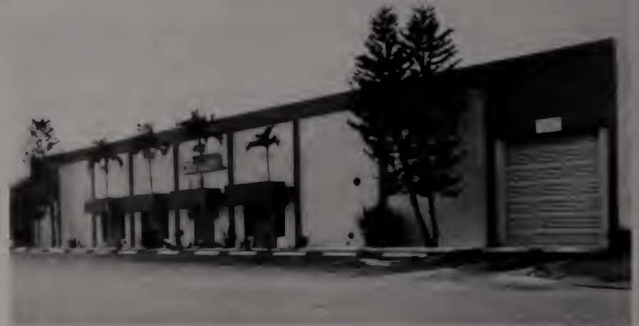
AWARD WINNER — Centuri Inc.'s offices and plant pictured above at 245 West 74 Place in Hialeah, Fla. has won an industrial landscaping award from the city's Beautification and Environmental Control Board.
