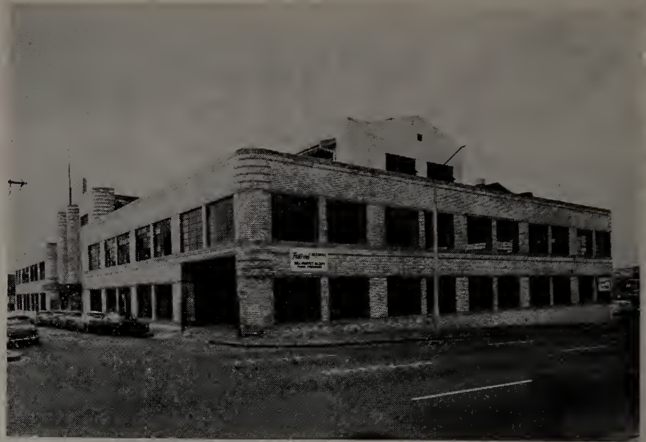
FOUND A NEW HOME —Here's a view of the new home for Festival Records Pty., Ltd. in Pymont, New South Wales. The building houses administrative offices and studios in addition to processing equipment and a pressing plant. Festival represents several American diskeries, including ABC, Atlantic, Liberty, Decca, UA, Dot, Monument, A&M, and Project 3.
