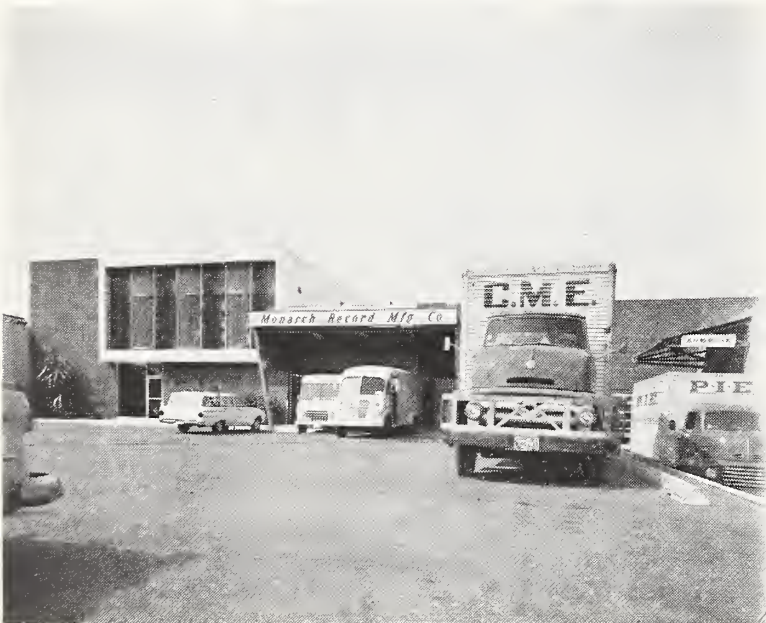
1. View of one of Monarch's buildings, showing loading area and entrance to offices.
