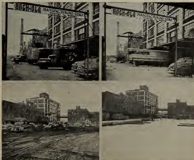
TOP—Receiving and Shipping. (l.) before, (r.) after.
