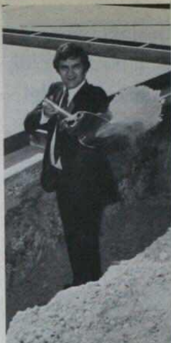
Dom Saccacio, Audio Magnetics president, turns over new shovel—and symbolic new leaf for company—at last month's groundbreaking ceremony for expanded Irvine, Calif., manufacturing plant.
