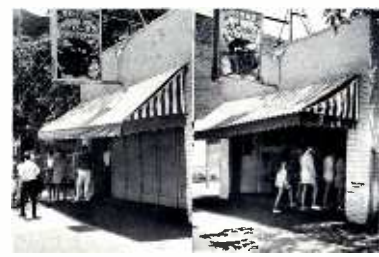
SLIDING DOOR (partially closed at left) opens to expose the entire front of the store.
