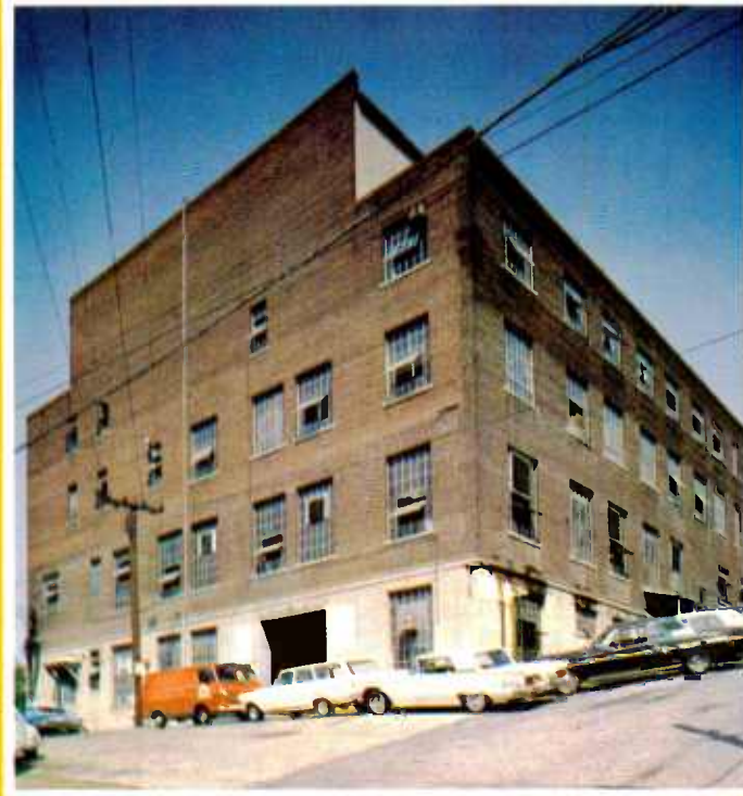
45,000 square feet sprinklered fire proof building — 2 hours from New York City.
