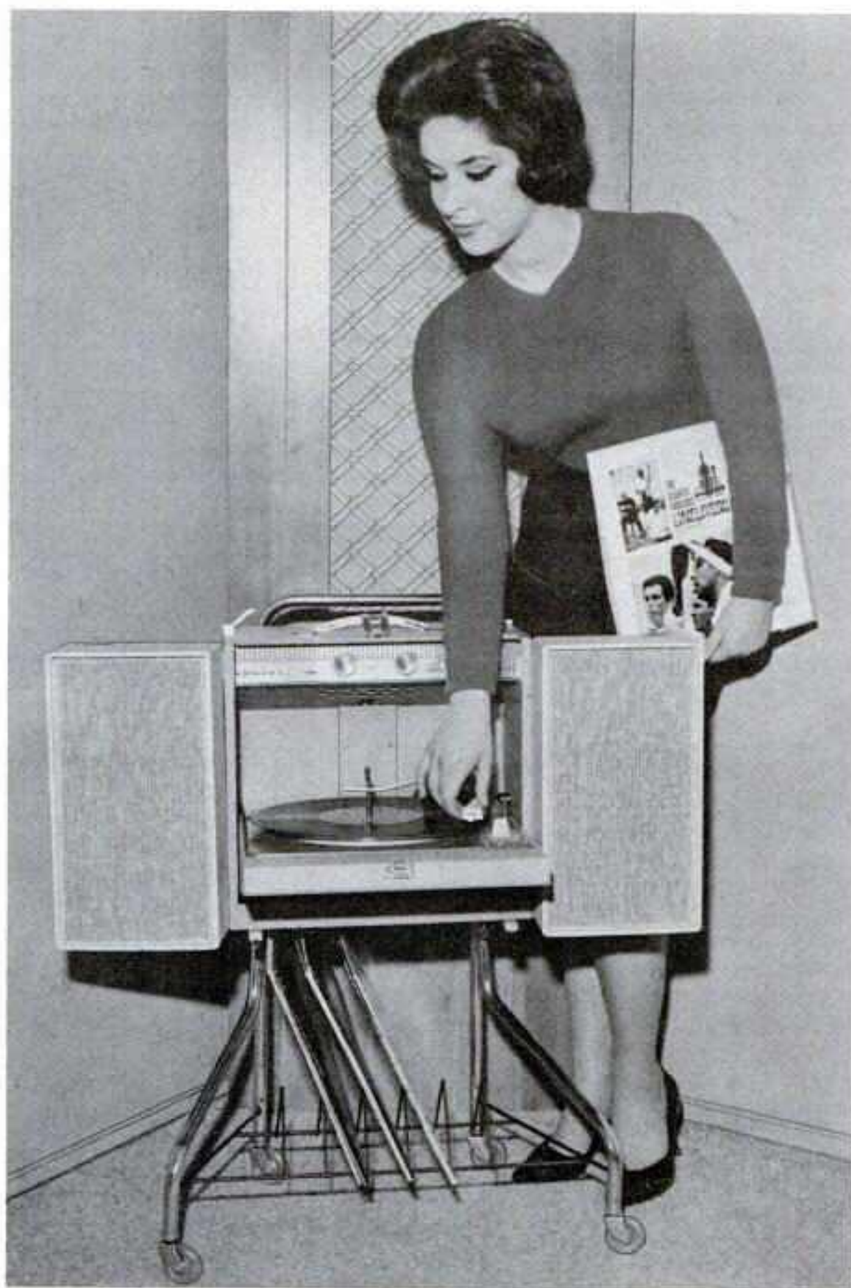
ATTRACTIVE MODEL is shown demonstrating the new Mardi Gras Admiral portable stereo phone. The slim unit is less than eight inches deep and the changer employs the modern, compact, tilt-out design. Hinged wing speakers may be detached and placed up to 24 feet apart. Suggested list is $79.95.
