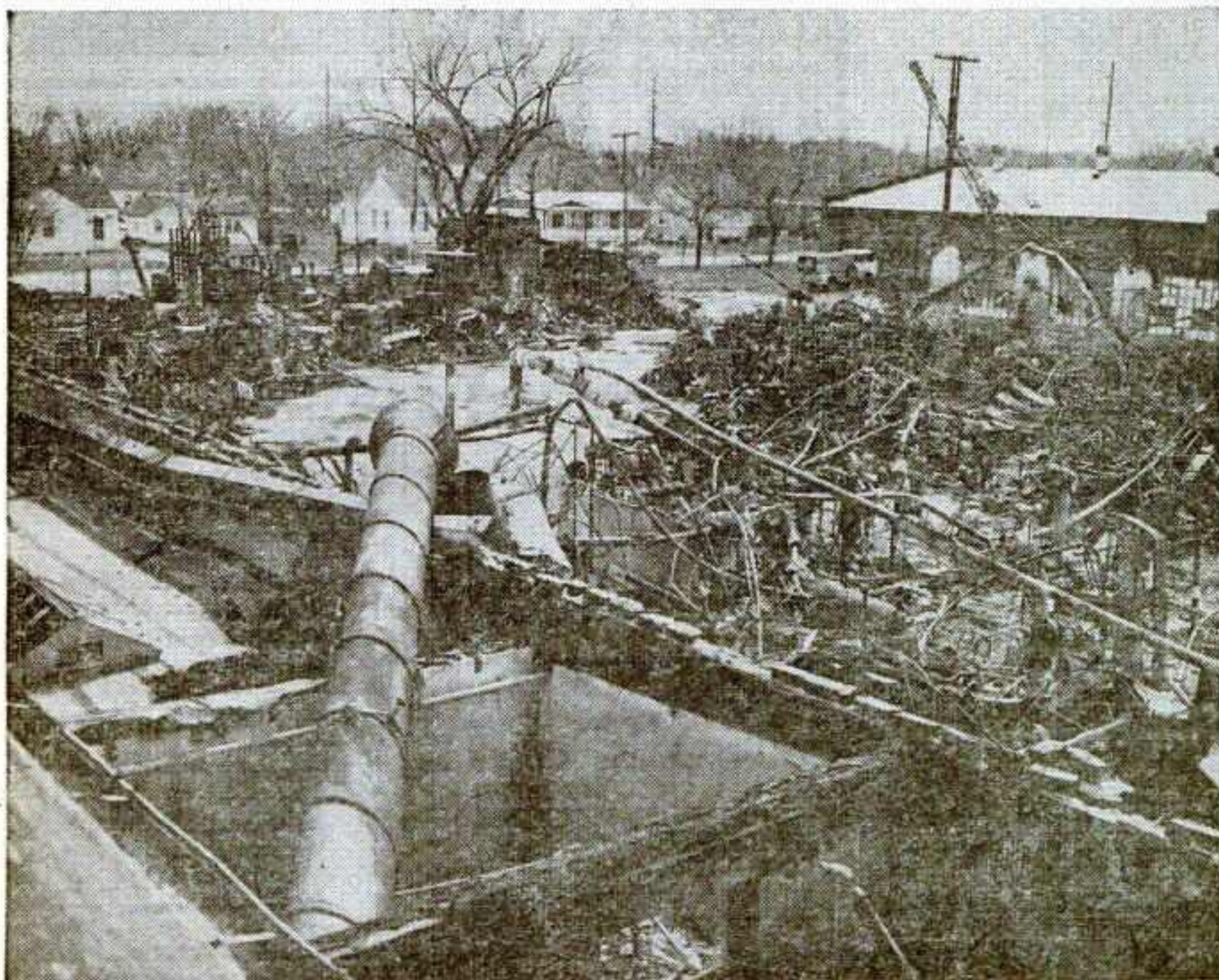
RESEMBLING A WAR-TORN AREA, the front of the Northwestern plant shows little left but skeletons of the buildings, machines and the factory's chimney after the smoke and fire cleared last April.
