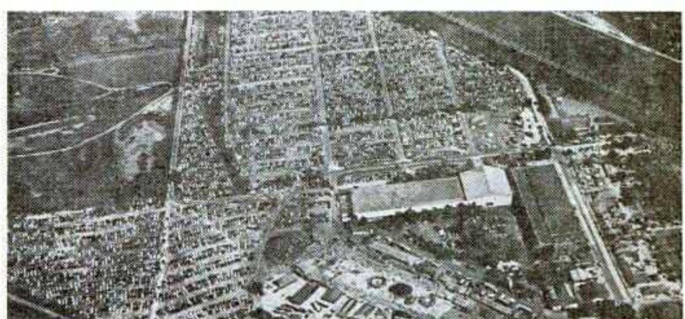
Aerial view of huge all-weather paved road parking area where more than 13,000 cars can be handled.
