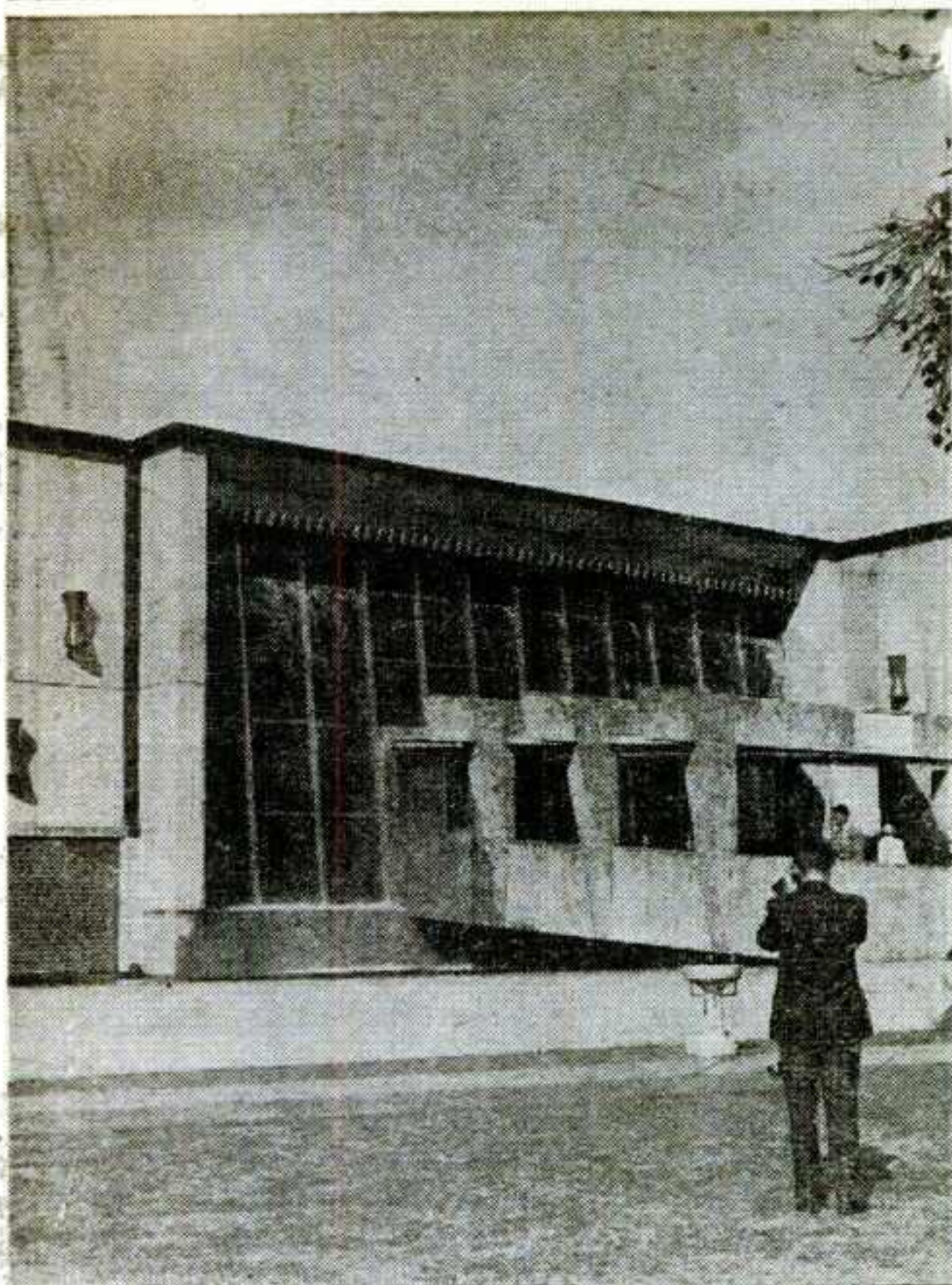
Water falls at two ends of the CNE's Food Products Building are crowd-stopping and provide a feeling of coolness and spaciousness to the interior. Colored lights played against the water add to the eye-catching qualities.
