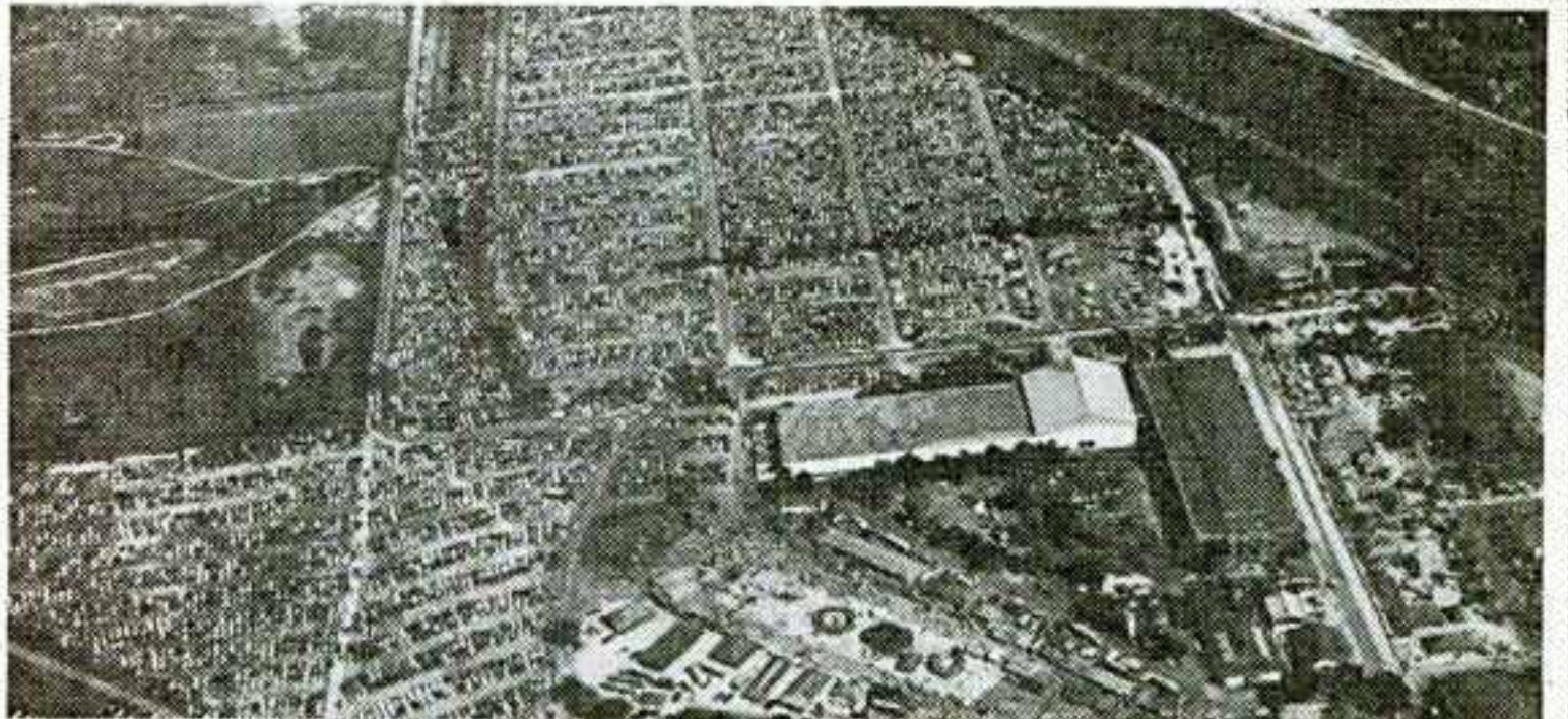
Aerial view of huge all-weather paved road parking area where more than 13,000 cars can be handled.
