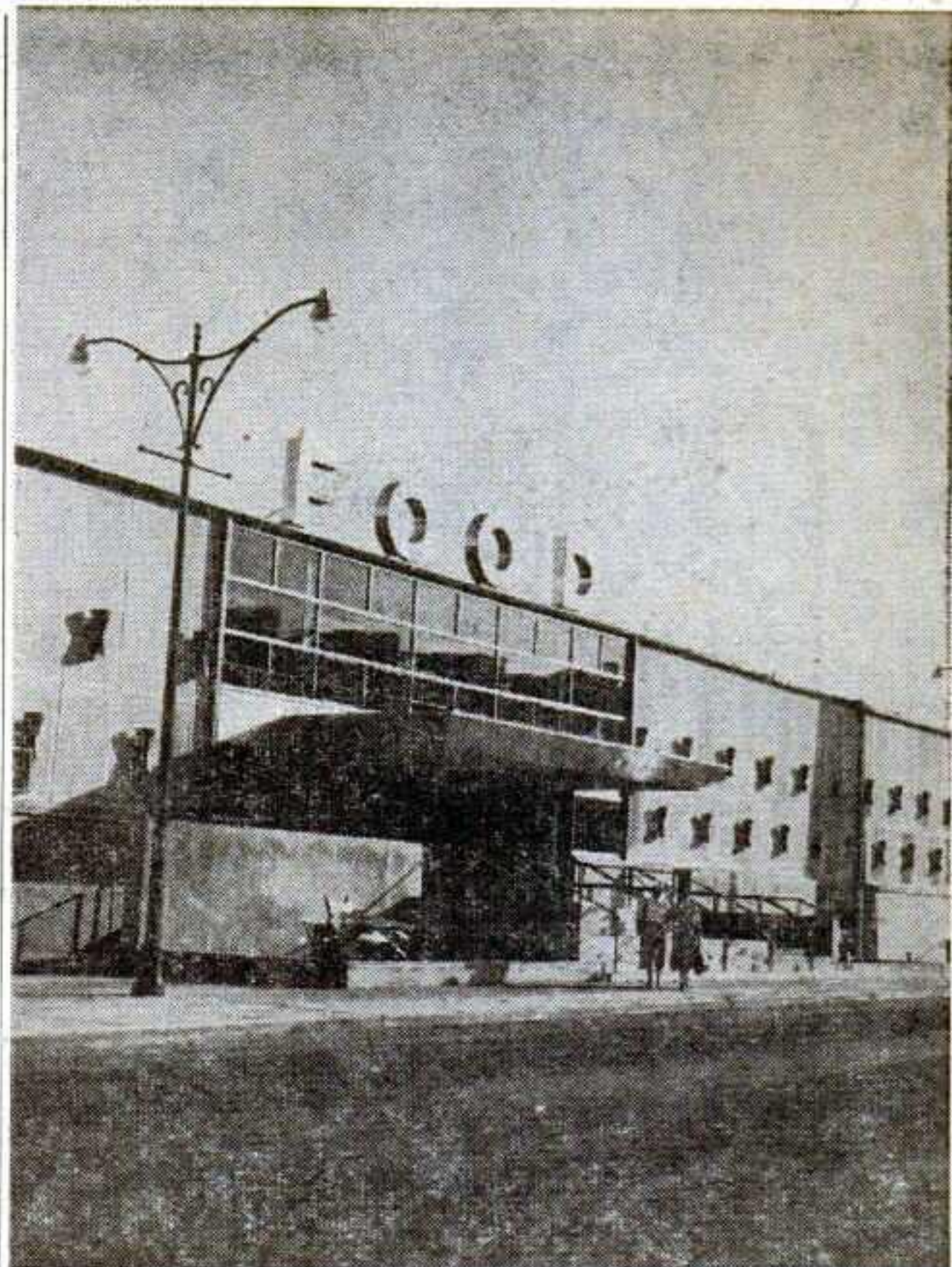
Simple, clean lines, a steel entrance canopy, an 80-foot pylon, blue-tinted glass in mezzanine windows, and screened lights give the new Foods Products Building at the Canadian National Exhibition an arresting front.
