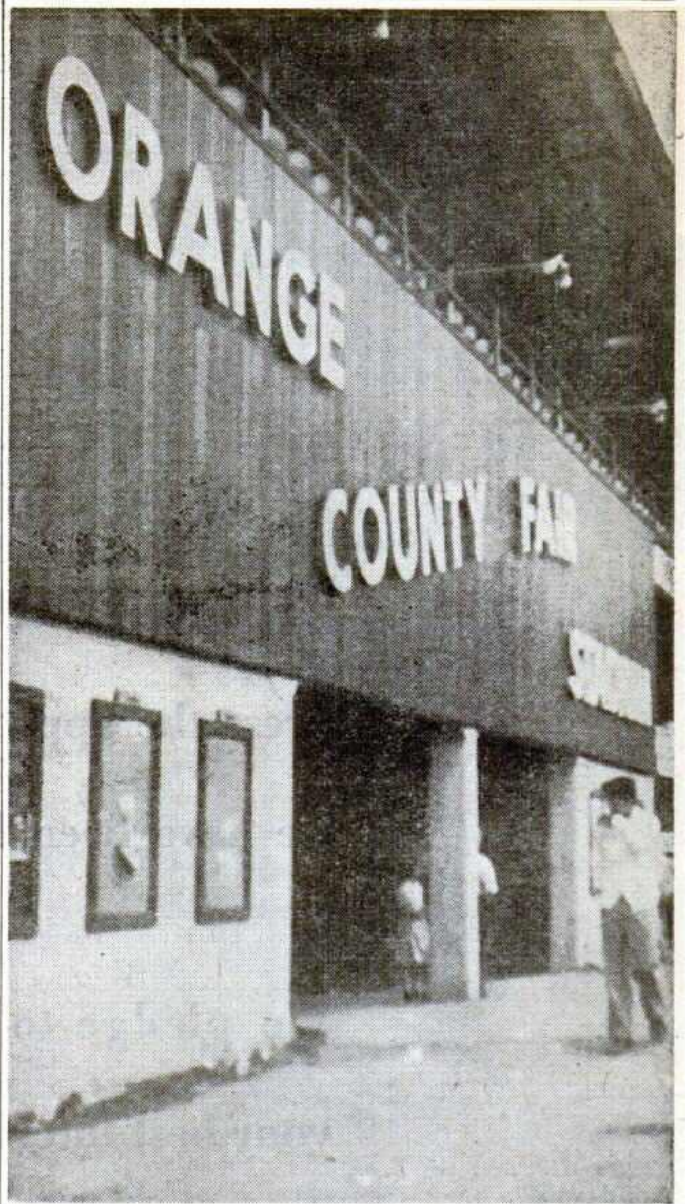
Given a new redwood face, with large cut-out letters, the grandstand at the 1954 Orange County Fair at Middletown, N. Y., was a sharp contrast to the old front which long had been an eyesore. The grandstand face-lifting is one of many projects planned to modernize the plant of the 114-year-old fair.
