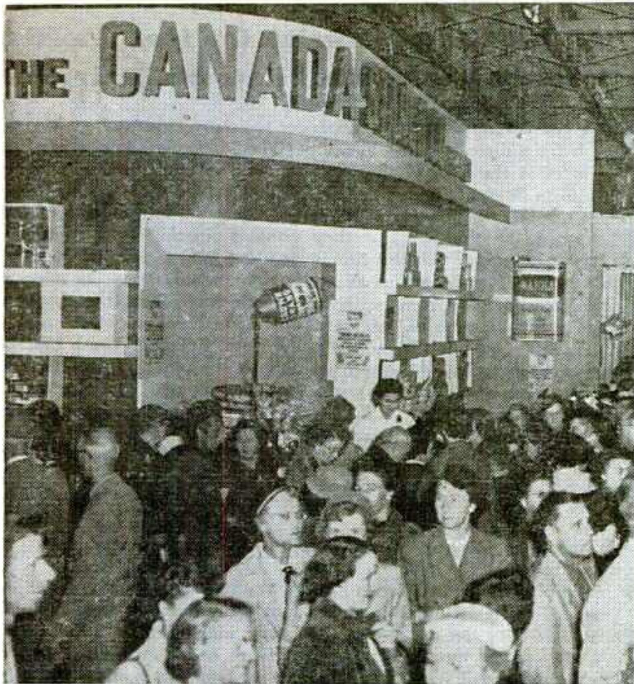
Slim-line fluorescent lights give excellent illumination. Exposed bar joists were some of the cost-cutting which enabled the CNE to erect the structure for $1,500,000.
