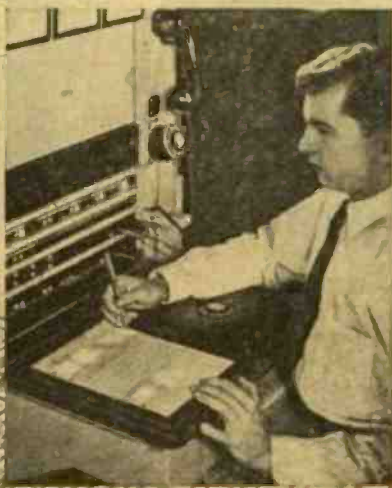
A pattern of lights on the chart gives this maintenance technician a complete report on the condition of control cable circuit. Chart is shown below.
