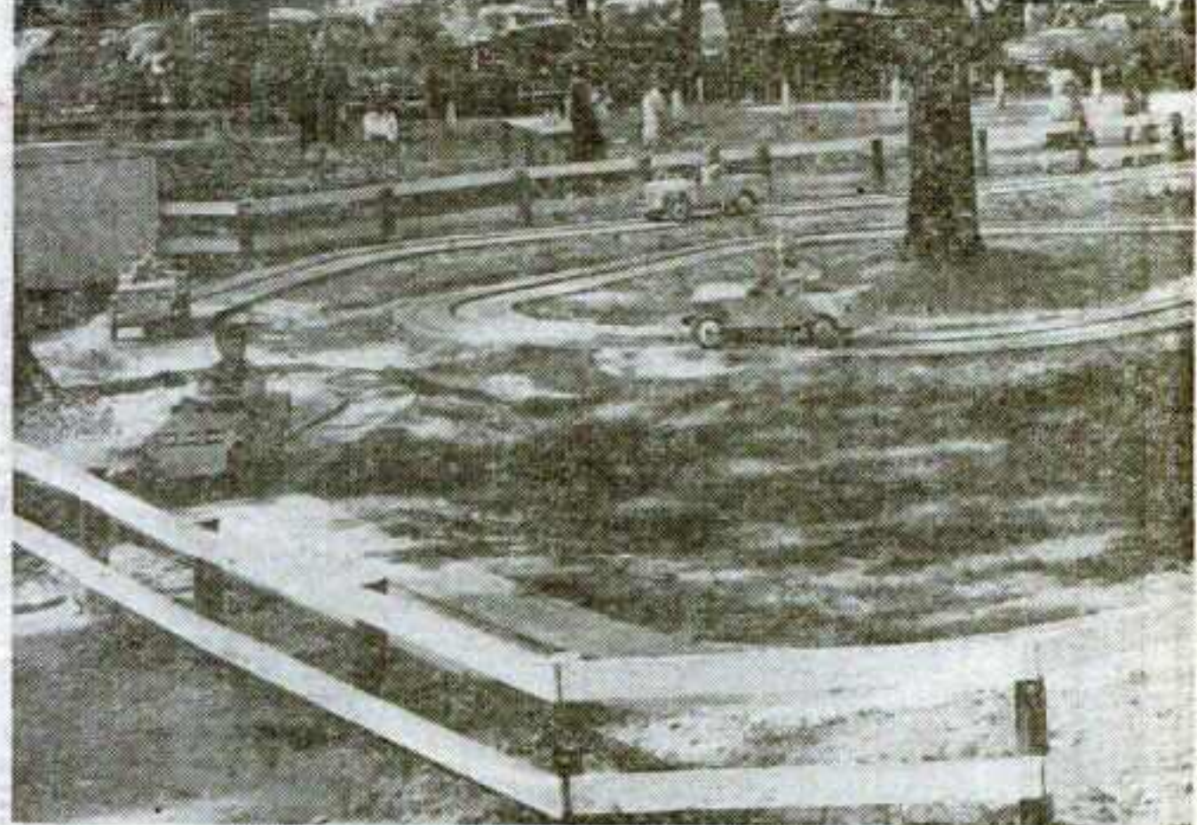
JEEP RIDE "down the highway" for the kids. "The cutest ride you ever saw" appeals to parents and children alike. A non-circular auto ride in sturdy, well-engineered jeeps powered by storage batteries, built to stand rough usage. Will run for 4 to 6 hours steady. Batteries can be recharged over night. 5 Autos, one around every minute, means 60 trips per hour per car, 300 fares per hour capacity. Top Kiddieland money-maker at New Toledo Beach.
