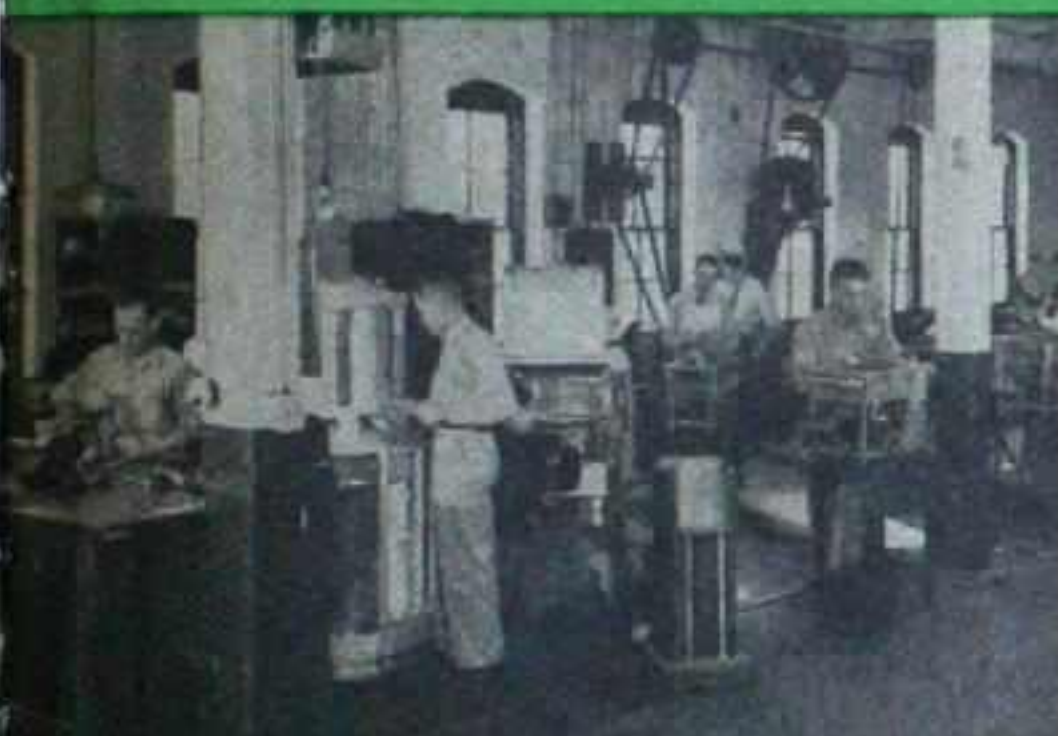
MECHANISMS—CLEANED, REPAIRED AND ADJUSTED
