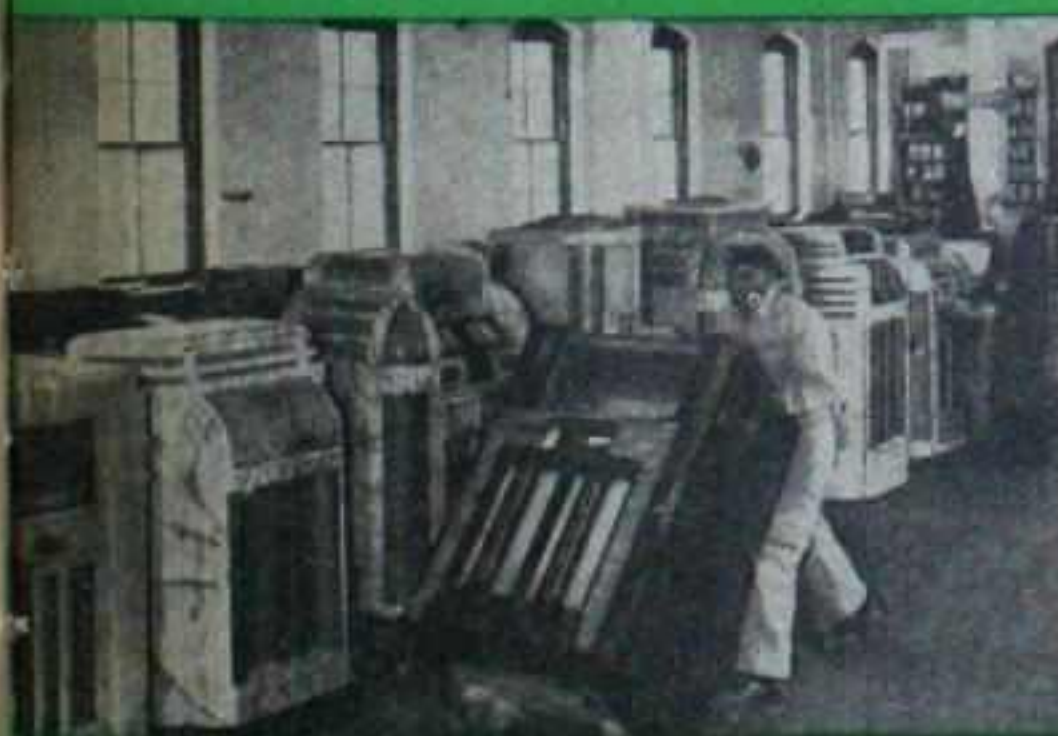
INCOMING CABINETS RECEIVED FOR REFINISHING
